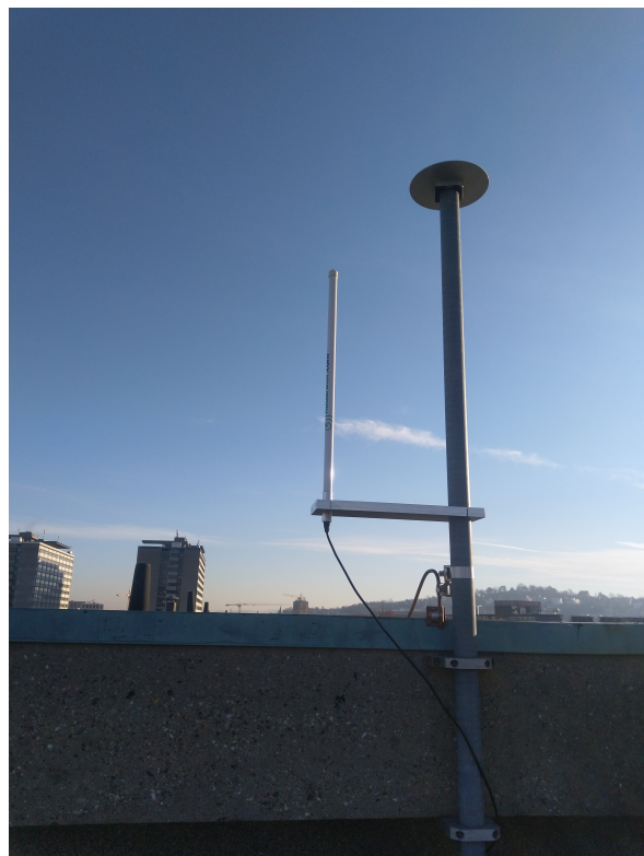
Figure 4: ADS-B antenna on the roof of the building of the institutes building.
